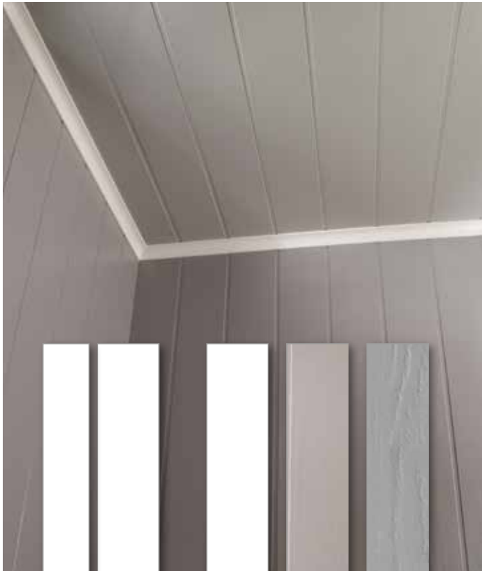
Wood Single panel Skygge installed on wall and Mist in the ceiling
